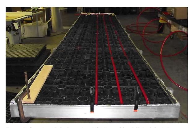
**Figure 05**: The bottom layer of Endura-Form panels are laid in the tray and the task of fitting the heating lines starts. The lower layer of panels are fitted with fixed receiving nuts for secure fastening of the top panel layer. The bottom panels are also fitted with drain holes (100 per panel) to allow proper drainage of the interior of the panel assembly.
