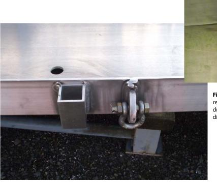
**Figure 02**: A closer view of the railing post socket, the lifting lug and shackle and one of the drain holes. The side is 4" high. There are four lifting lugs and shackles are 2.5 ton capacity and has a cotter pinned nut and bolt. Total weight of the completed 20' walkway is less than 1000 lbs.
