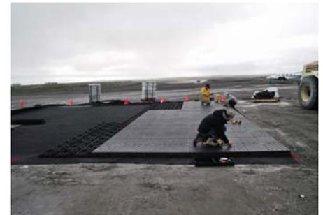
The layout of the Endura-Form panels starts over top a layer of material.
